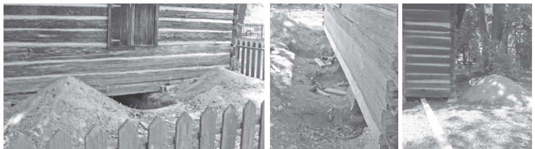
Below: Photos of the current repair project which involves digging underneath the cabin.
