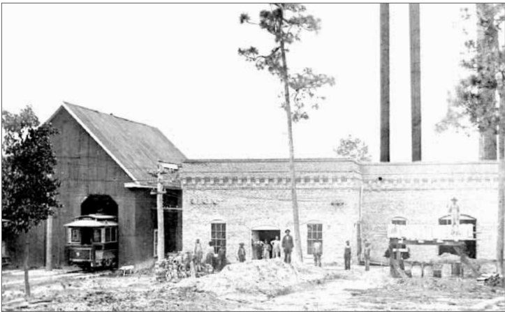
Trolley Barn to left of Pinehurst Power Plant. Now the Pinehurst Brewery.
