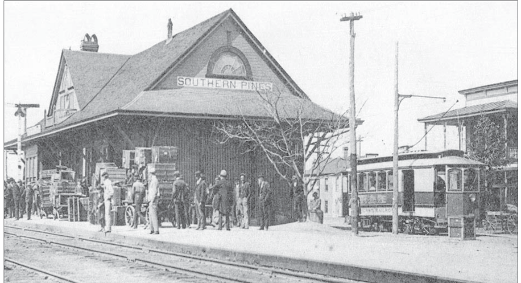
Tufts Trolley at Southern Pines Depot.
