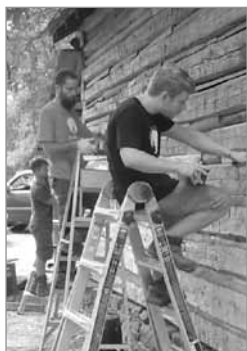
Tobacco Barn Restoration - Ted Lawrence who originally restored the Barn with son Thad Lawrence and Josh Smith of N.C. Cedar who did the current restoration. (Left) the men "daubing" between the logs to seal the structure.
