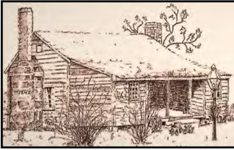
Shaw House, Garner House, Sanders Cabin & Tobacco Barn in Southern Pines
